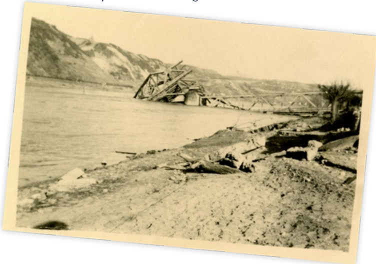
DESTROYED REMAGEN BRIDGE, GERMANY, 1945. THE BRIDGE COLLAPSED 10 DAYS AFTER ITS CAPTURE, BUT BY THAT TIME OTHER CROSSINGS HAD BEEN ESTABLISHED ACROSS THE RHINE. FROM THE COLLECTION OF THE NATIONAL WWII MUSEUM, 2013.297.236_1
