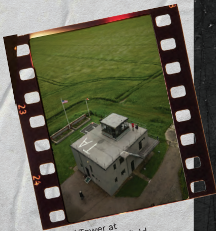
Control Tower at Thorpe Abbotts Airfield
